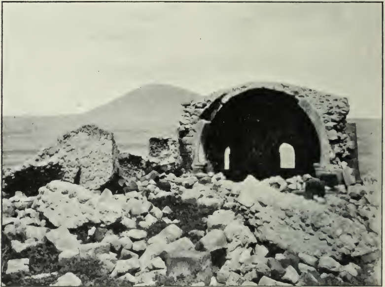
FIG. 35.—No. 6, interior of apse.
